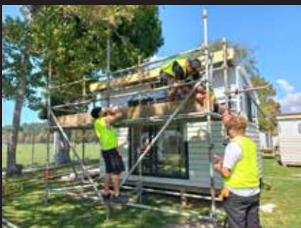
The construction team erecting the scaffold
