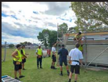
The construction team installing the scaffold with Beaver
