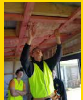
Cole Hati installing the insulation
